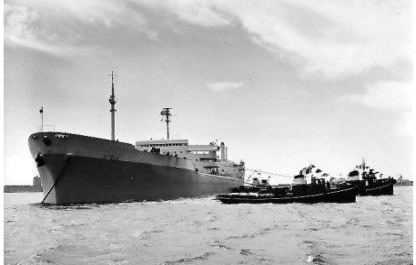
The ship is 259 meters long, 35,6 meters wide (almost two meters more than the cruise liner *France...*), 18,40 meters deep and her draught can reach 13,87 meters. She is propelled by two turbines totaling 24,000 horsepower at the speed of 16,5 knots.
