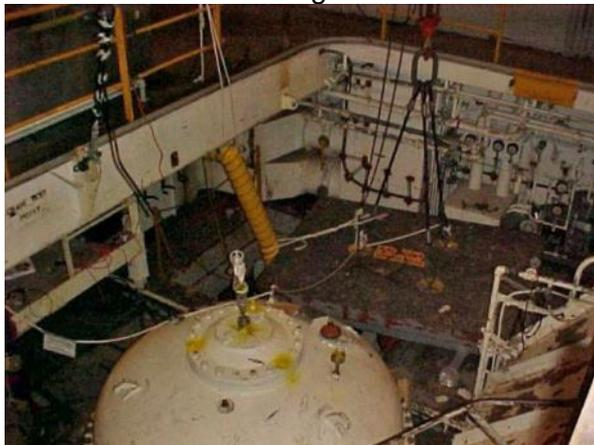
Refueling Room aboard *Sturgis*, showing Spent Fuel Tank Lid and Access Plug. (Corps Photo)
